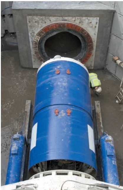
Typical pipe jacking eyes (see note (g) on page 18 opposite)
