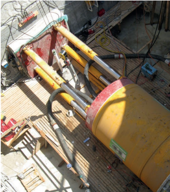
Thrust pit set-up
